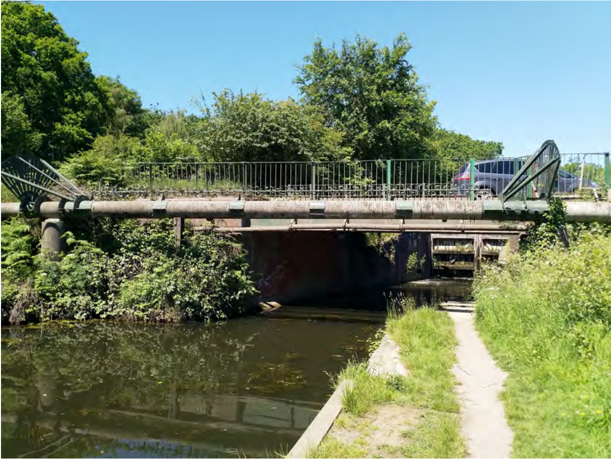
Image 25—View Looking North West towards Government Road Bridge and Ash Lock beyond
