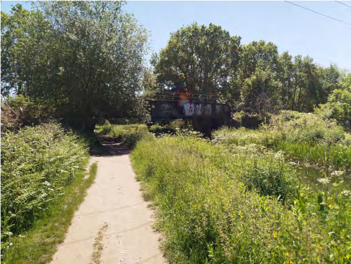
Image 26— View looking South east from Government Road Bridge towards the railway bridge
